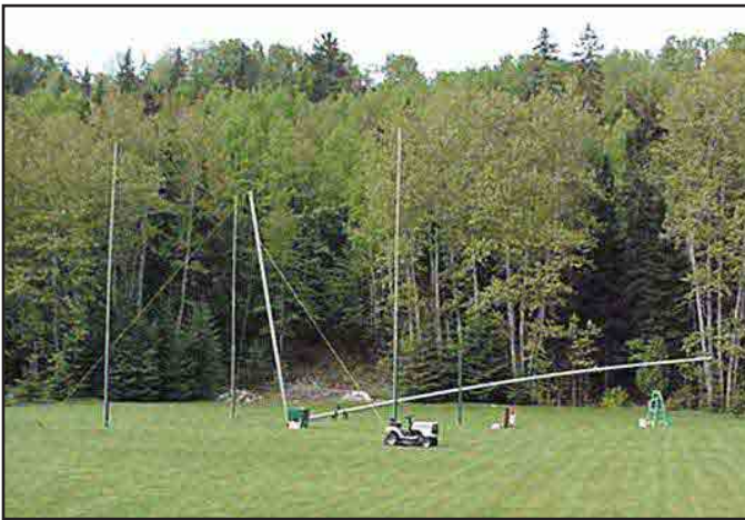
Figure 10—Layout of derrick for raising the element. L1=the length of the derrick boom. L2=L1. L3=any length greater than L2.
