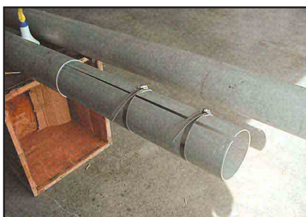
Figure 2—The doubler ready for insertion into the main section.
