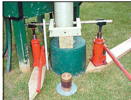
Figure 12—Two views of the pivot fixture for positioning the base insulator.
