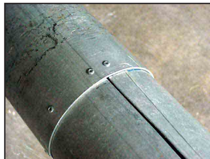
Figure 3—The doubler riveted into place.
